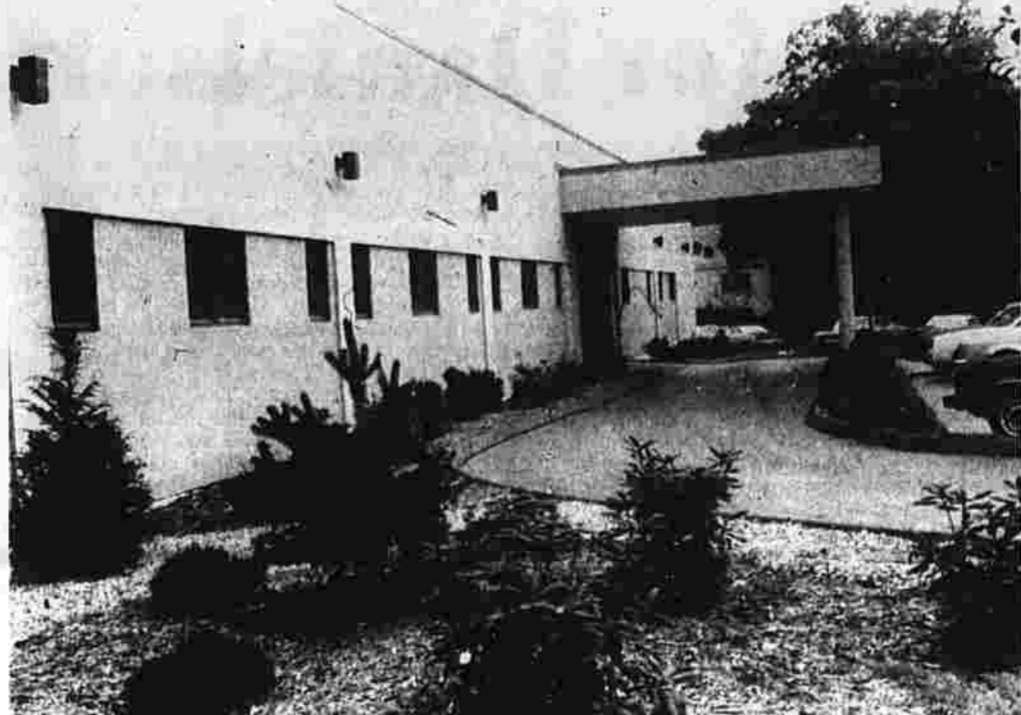
The physicians who planned and carried out the renovation of the former A & P building, with portico, is surrounded by building on East Center Street, were presented this week with the beautification award, by the Greater Manchester Chamber of Commerce.
